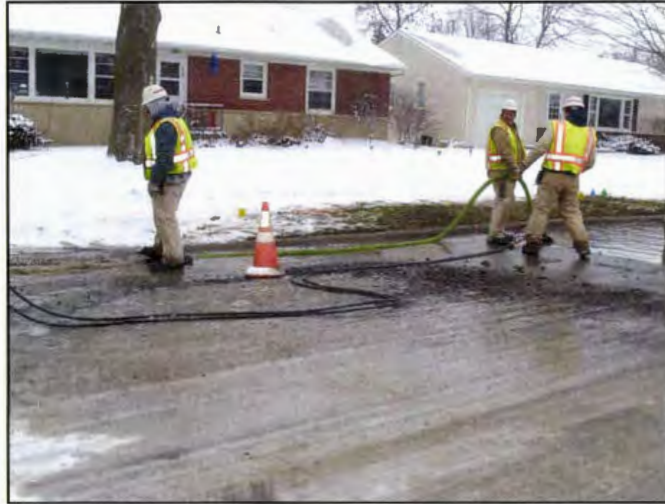
Figure 35. Dewatering the trench.
