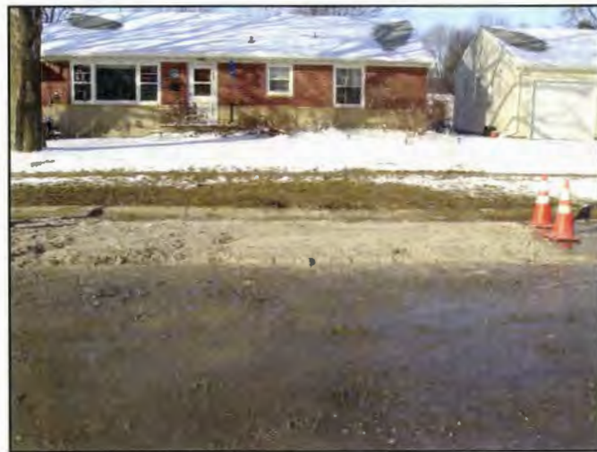
Figure 39. Trench ready for cold patch.
