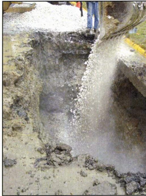
Figure 27. Bedding material dumped into trench.
