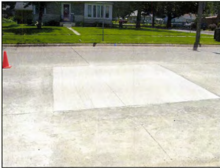
Figure 50. Completed surface in Des Moines.
