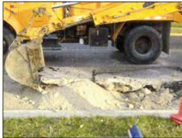
Figure 58. Pavement removal.
