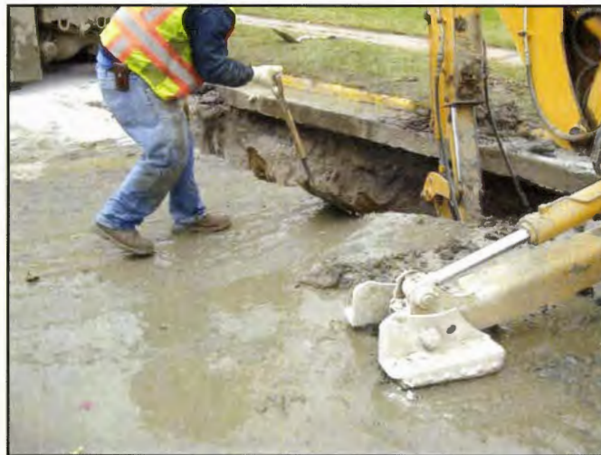
Figure 29. Saturated material shoveled into the trench.
