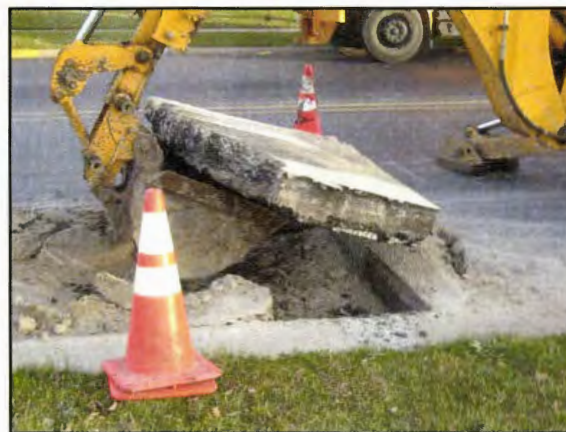
Figure 31. Pavement removal.
