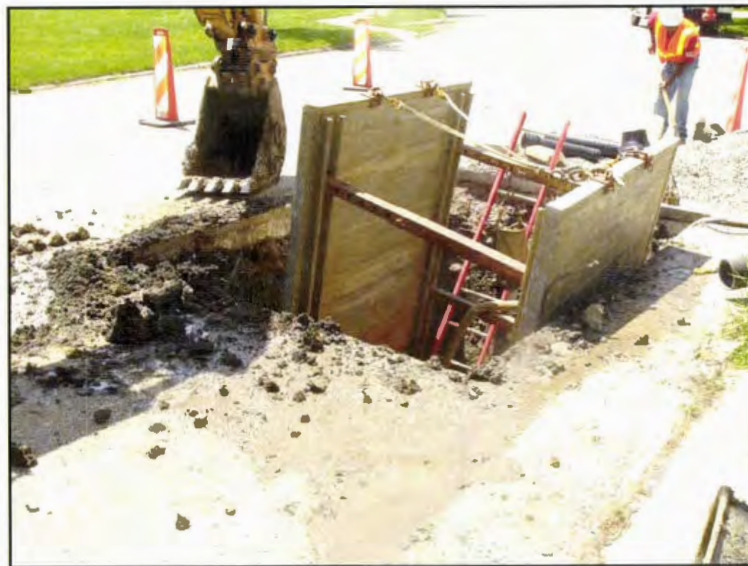
Figure 40. Shoring box in place.
