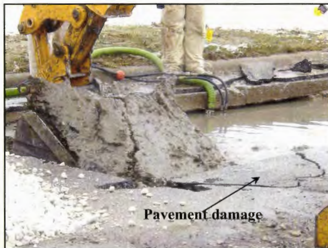
Figure 36. Saturated material being excavated.
