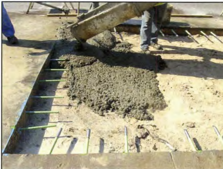
Figure 49. Concrete placement in Des Moines.
