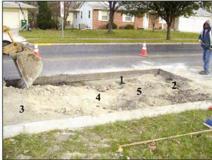
Figure 59. Testing layout of trench.
