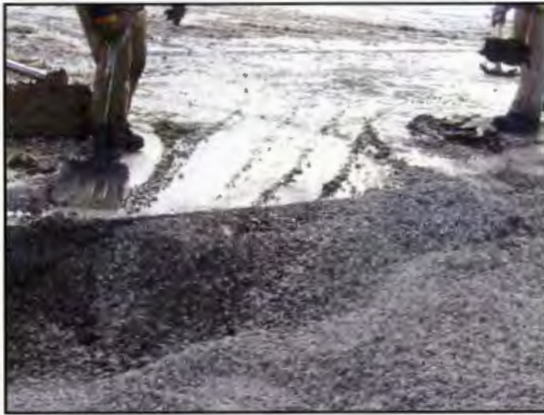
a) Cleaning excess material into the trench
