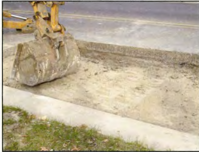
Figure 32. Backhoe bucket compaction.
