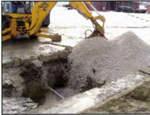
a) Pushing in backfill material
