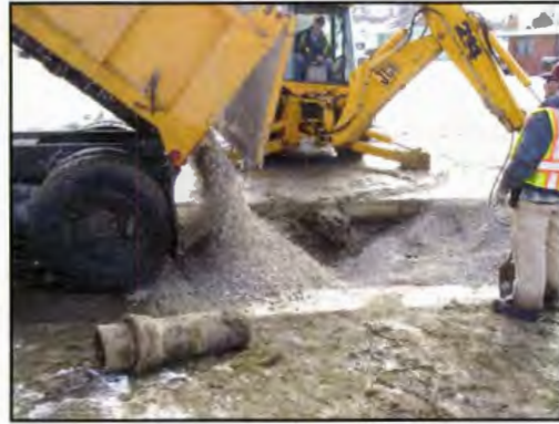
b) Dumping backfill material
