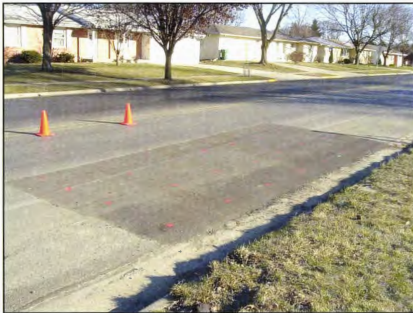
Figure 33. Ames site completed.
