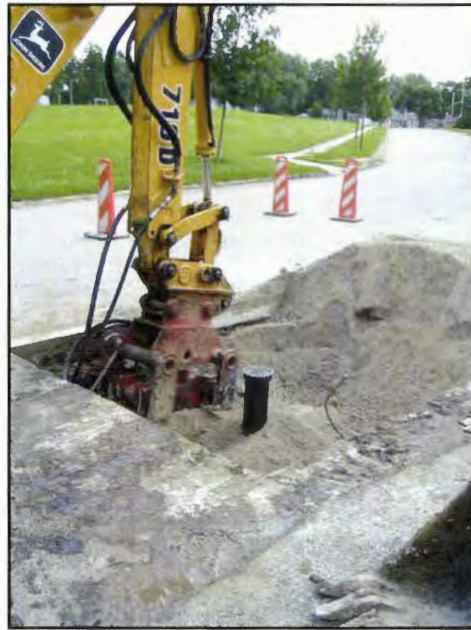
Figure 41. Backfill compacted into trench.
