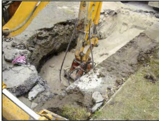
Figure 28. Compaction of backfill material.
