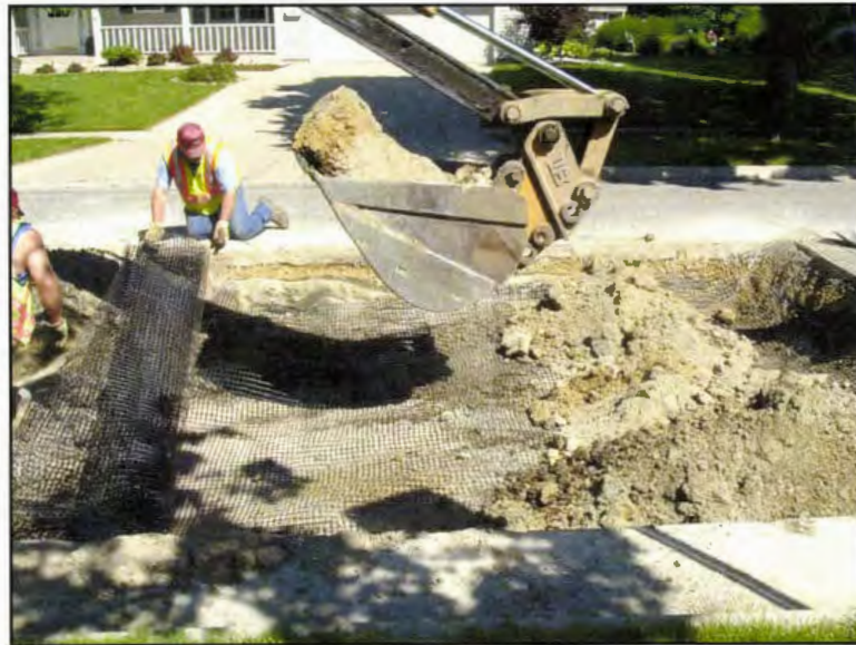
Figure 95. Geogrid being placed.
