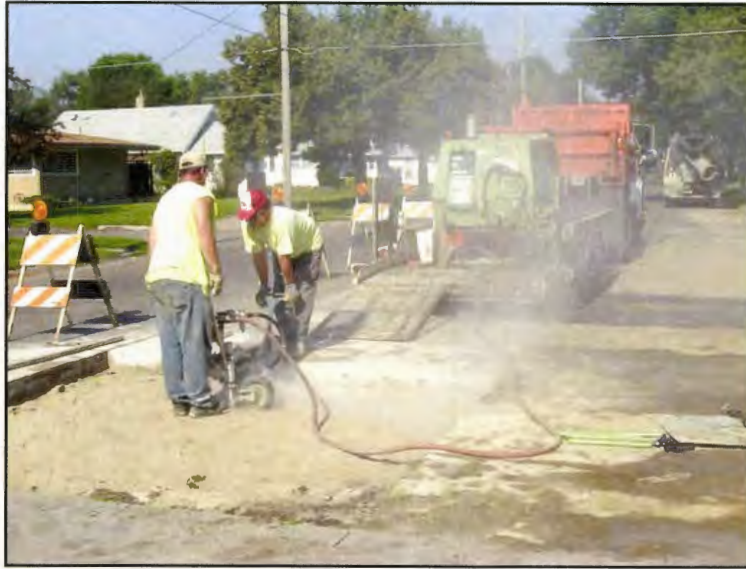
Figure 48. Drilling spacings for dowel bars.
