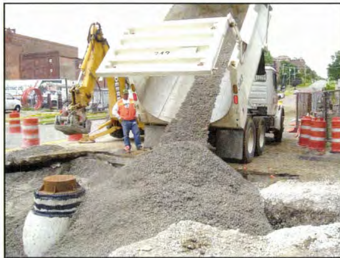
Figure 43. Large backfill lift being placed.
