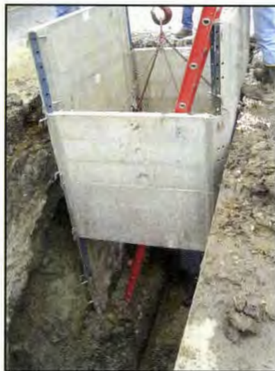
Figure 26. Shoring box placed into trench.
