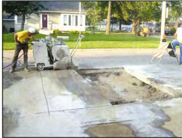
Figure 46. Concrete pavement cut being made.
