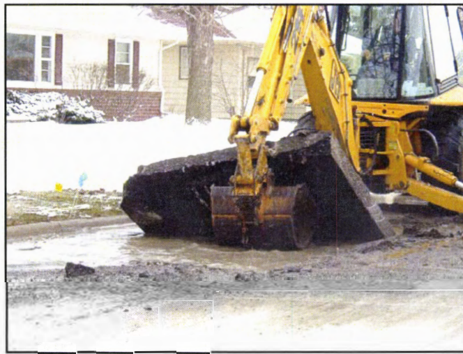
Figure 34. Pavement removal from Ames winter break site.
